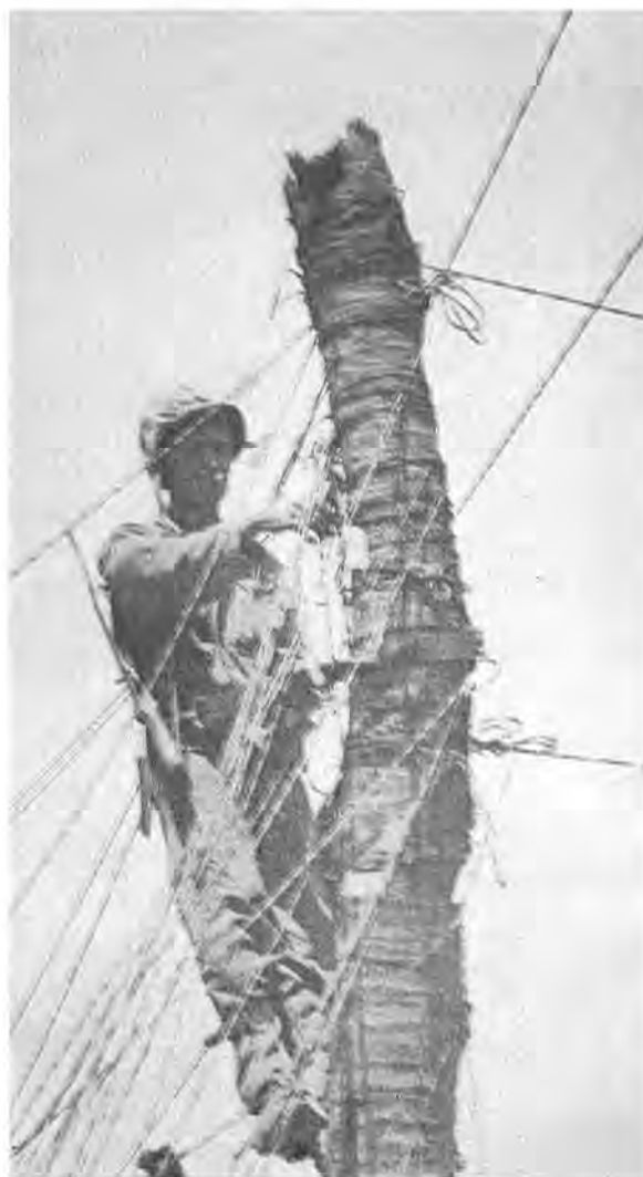
COMMUNICATORS raised their wires from the ground to makeshift telephone poles when the shooting quieted down.
