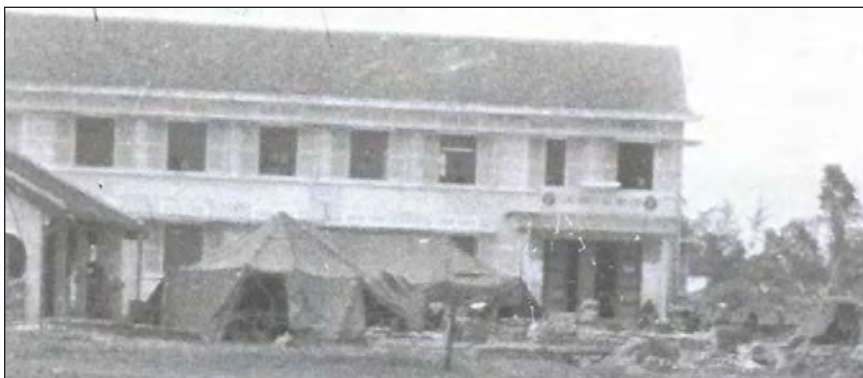
Figure 3.3. Construction of CAC compound at the Gia Le Hospital
