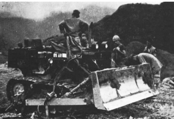
Engineer Marines use bulldozer to quickly construct fire base.
