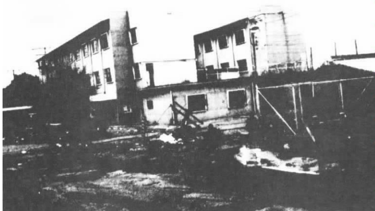
Landing zone in PX compound.
