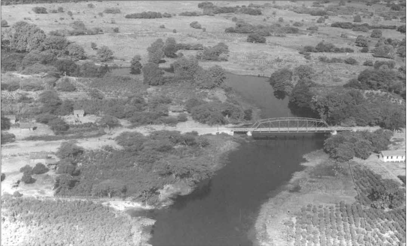
Official U.S. Marine Corps photo 51627, by 1stLt L. N. Bertol, Historical Reference Branch, Marine Corps History Division Haiti, October 1933. Iron bridge across the LaQuinte River, about 3 km from the town of Gonaïves, Haiti, one of the many bridges constructed in Haiti with an assist by U.S. Marine Corps forces and the Marine-trained Garde d'Haiti.
