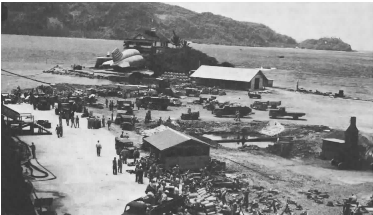
Barrage balloon in background ready in case of air attack on unloading area. (USMC Photo 51110)
