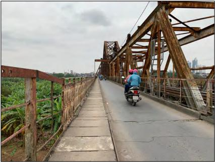
Looking southwest from the bridge. Junction of old and new bridge is seen where ornamental hand railing ends and repair begins. Crack along the road surface also shows the seam.
