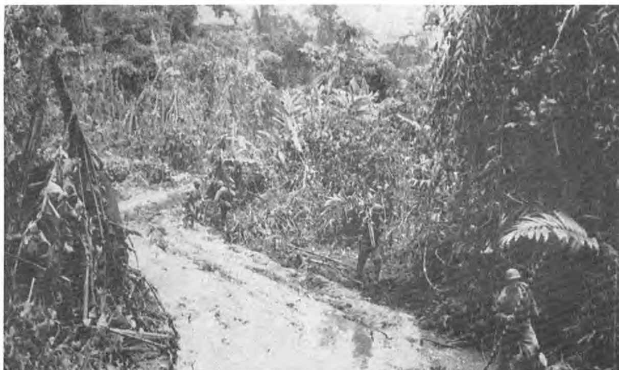
ENGINEERS MOVE UP ALONG A MUDDY TRAIL. Faced with swamp drainage, road building, airfield construction, and similar tasks, engineers played a vital part in the establishment of the advance base at Cape Torokina.
