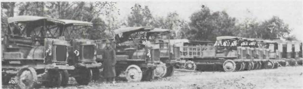
Jeffery Quad cargo trucks at Quantico in 1918. During the fall rains, the unpaved streets became a quagmire of mud that required the use of chains on the solid rubber-tired wheels. (USMC Photo 518095).
