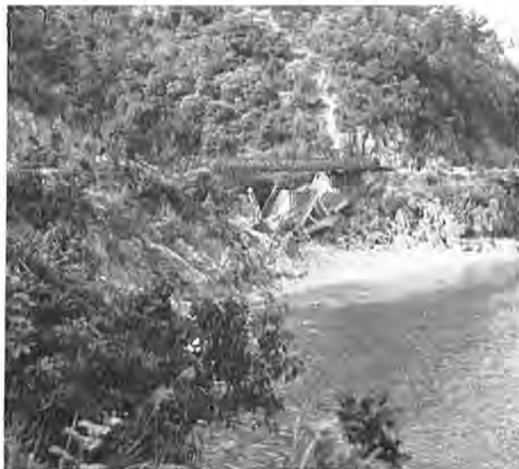
BAILEY BRIDGE erected by 6th Division engineers over the ruins of a bridge blown by the enemy in an attempt to block the drive into northern Okinawa.
