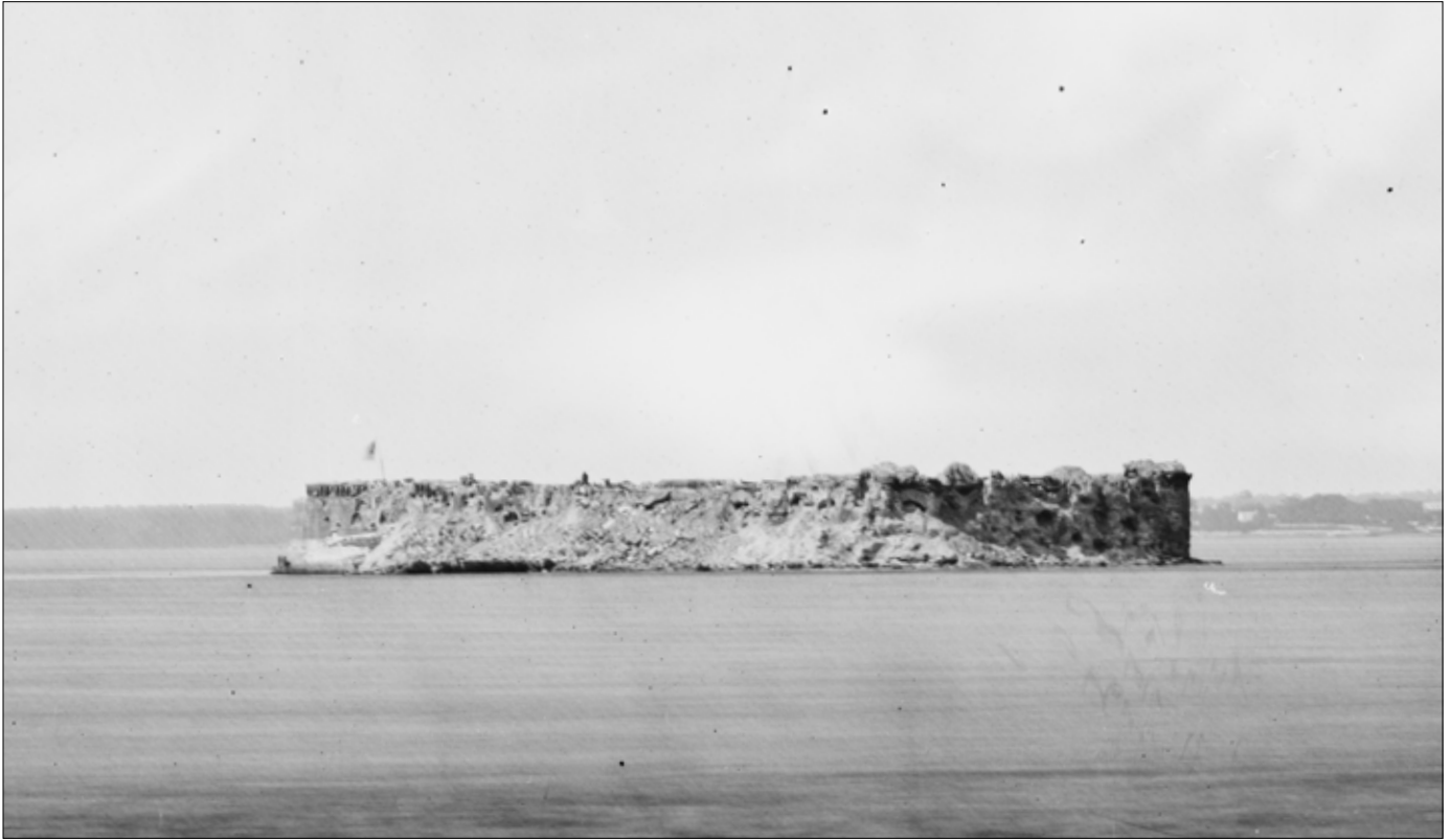
Photo by Haas and Peale, courtesy of Civil War Photographs, 1861–65 , Library of Congress, Prints and Photographs Division, call no. LC-B8156-43 A Fort Sumter, photographed on 23 August 1863, following the start of the Union bombardment. The large-caliber rounds from the Union artillery caused the fort's walls to crumble and created a roughly 45-degree ramp leading from the sea into the fort.
