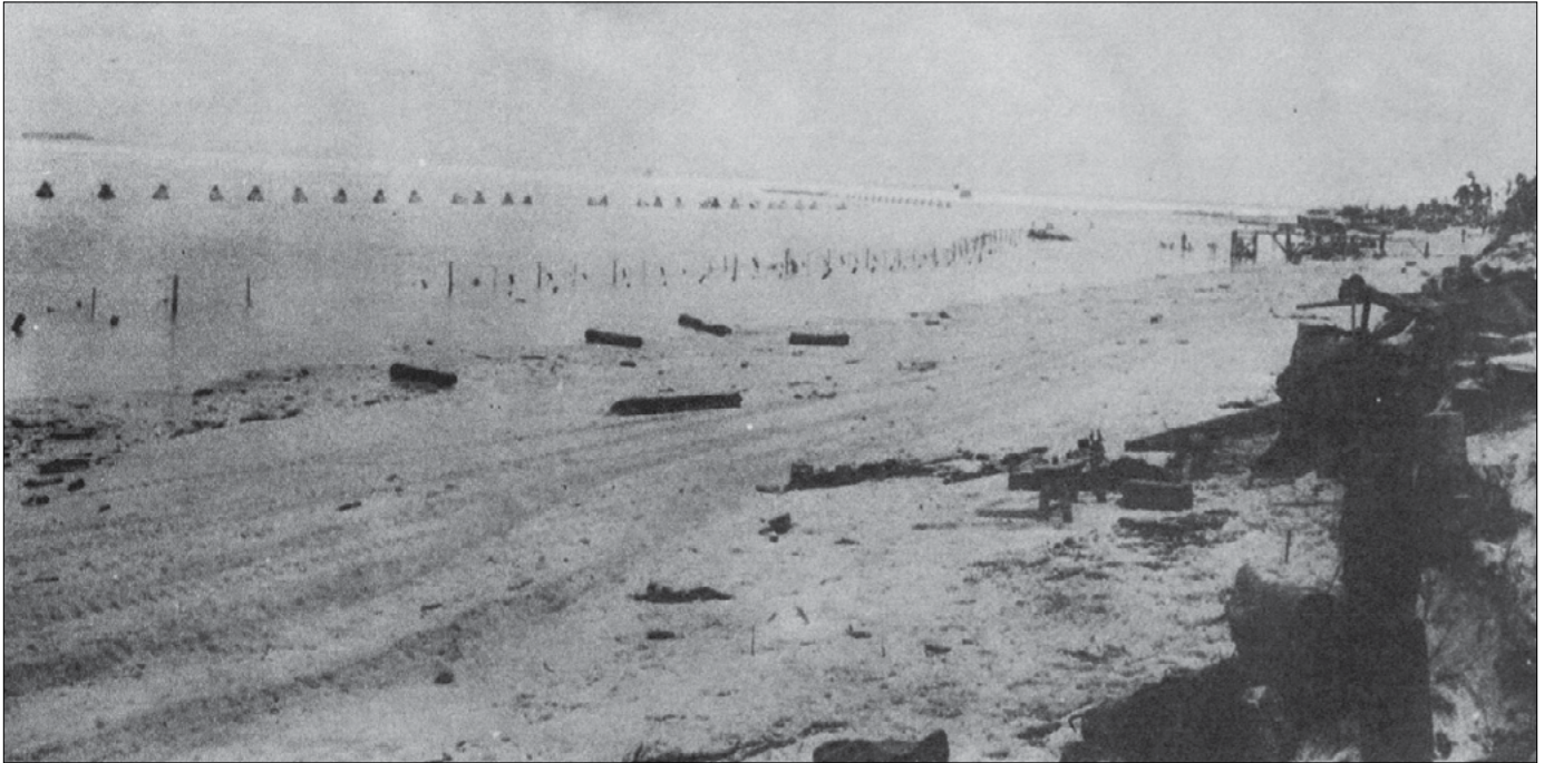
2d MarDiv Intelligence Section and POA Joint Intelligence Center, "Study of Japanese Defenses of Betio Island (Tarawa Atoll)," 170 Japanese obstacles on the western beach at Betio including tetrahedrons, wire, and a coconut log sea wall.
