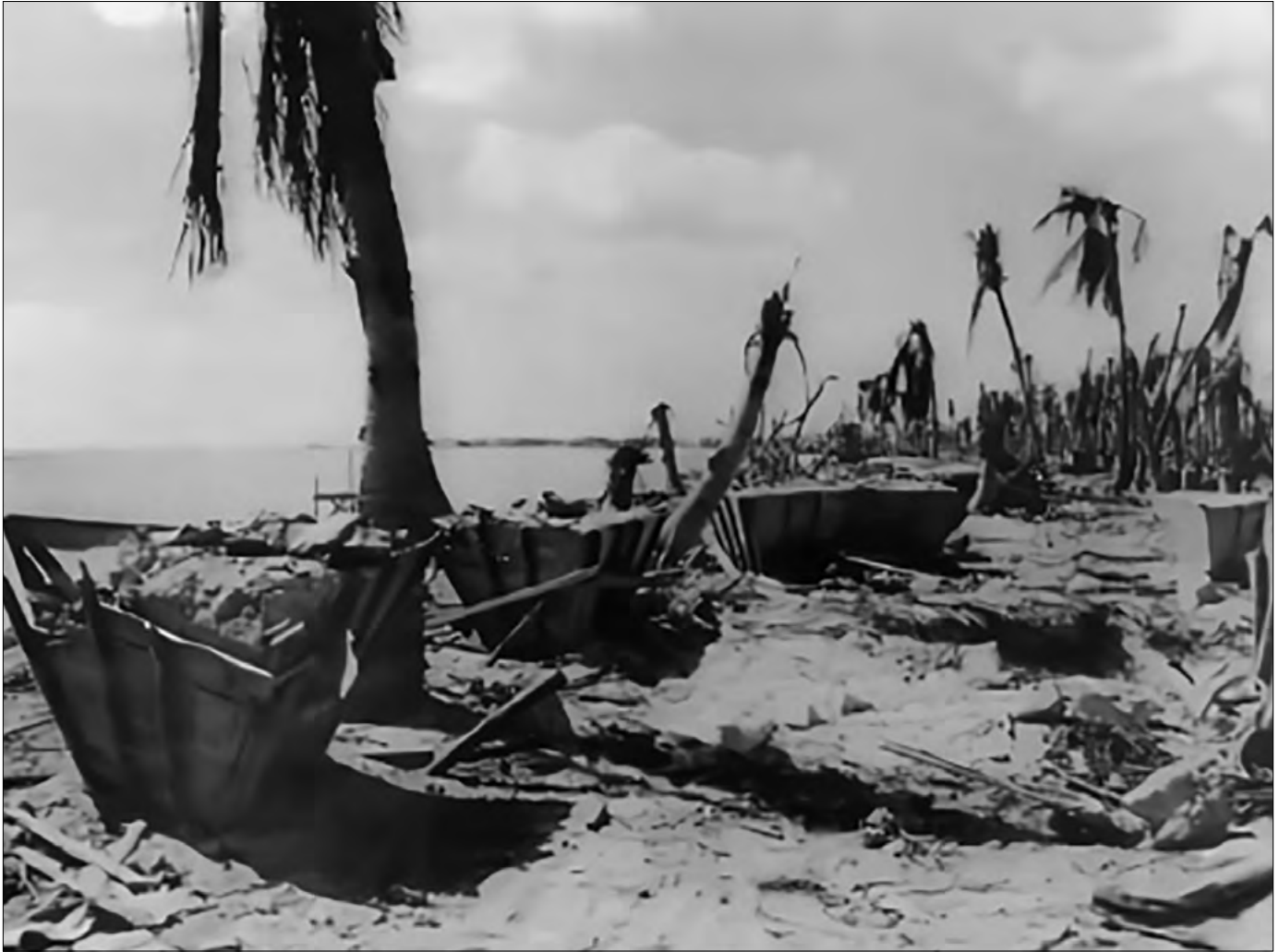
2d MarDiv Intelligence Section and POA Joint Intelligence Center, "Study of Japanese Defenses of Betio Island (Tarawa Atoll)," 171 Japanese tetrahedron molds at Tarawa.
