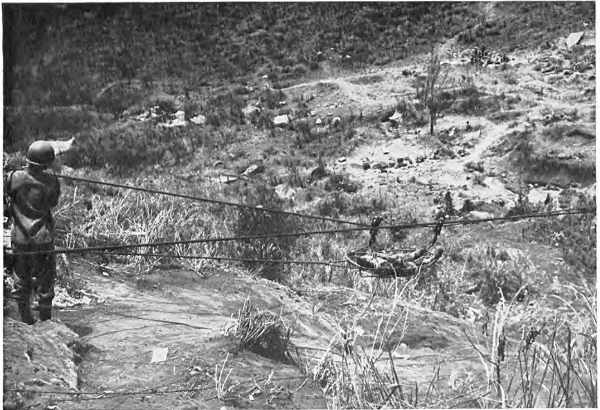
CABLE LIFT built by the 19th Marines used to evacuate casualties from the top of the steep cliff in the 21st Marines zone of action.
