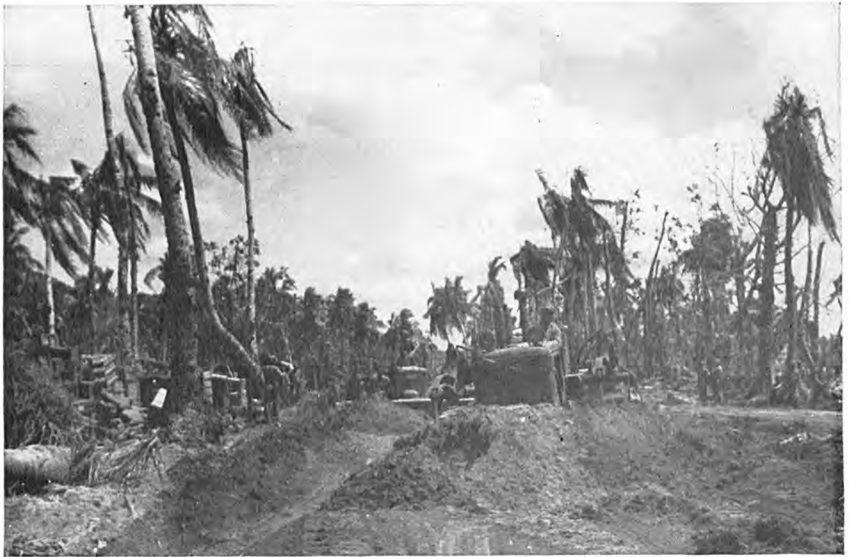
SEABEES on bulldozers prepare the bed of a new road linking the Agat Bay area with the IITAC front lines.
