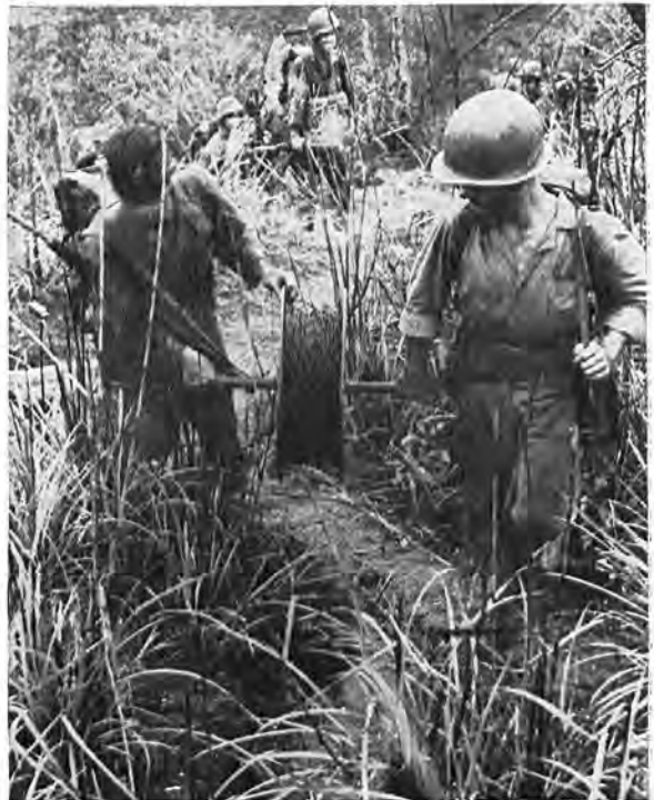
WIREMEN close behind assault troops lay a line to a forward command post.
