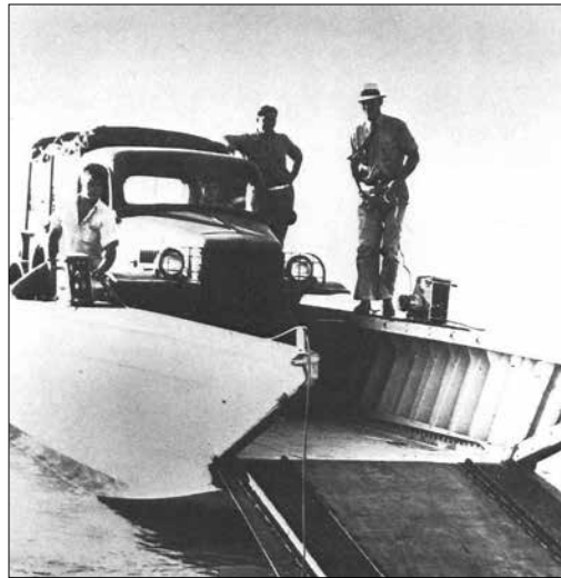
The design of this Higgins landing craft, loaded with a military truck, shown here in May 1941, served as the basis for the landing craft, vehicle and personnel (LCVP).
