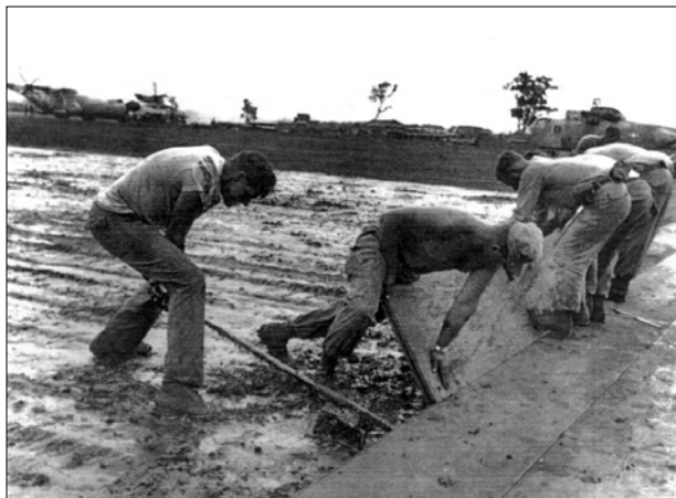
Seabees of Mobile Construction Battalion-301 set and seal aluminum runway mats into place at Khe Sanh Combat Base.
