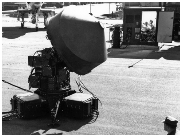
A static display of the AN/TPQ-10 system at Point Mugu, California, in 1962. In the foreground is the precision tracking radar and in the background on the right is the control van. The van was originally nicknamed a "beli-but" to emphasize that the entire system could be moved around the battlefield by helicopter. Inside the open door of the control van, two Marines of an Air Support Radar Team can be seen seated at the monitors, as they would be when guiding an aircraft to a computed release point to put its bombs on target. The static display also includes an A-4 in the background on the left, which is significant because the A-4 was designed only for bombing in daylight and permissive weather conditions. The TPQ-10, however, could be used to put a Skyhawk's bombs on target day or night, and in any kind of weather.
