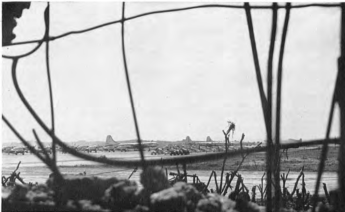
AFTER THE BATTLE twisted steel reinforcing rods form laticework through which B-29's and P-51's' are viewed from inside demolished Japanese blockhouse. (AF Photo)
