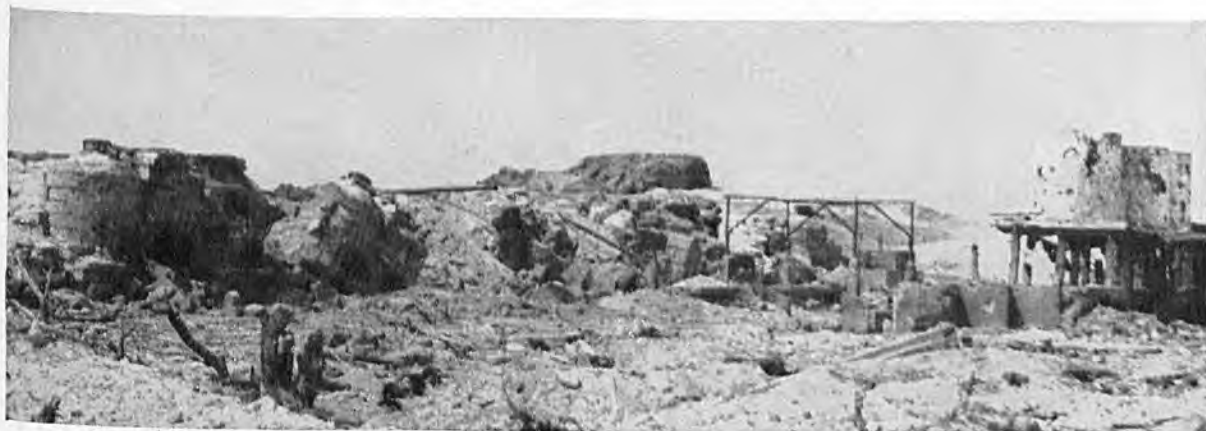
EVAPORATION VATS AND FURNACES located near the sulfur mines show destruction wrought on surface installations during the fierce fighting. This area is just west of Motoyama Village.
