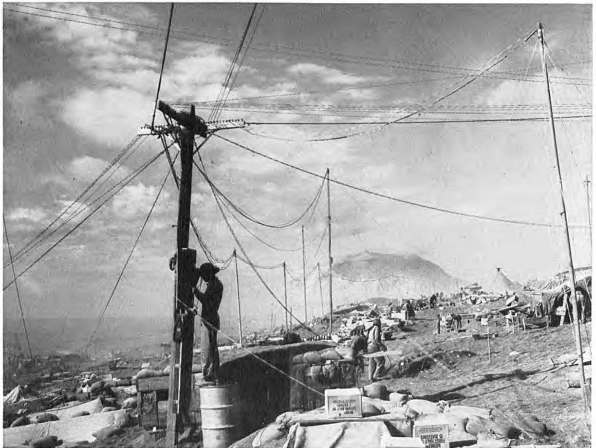
TELEPHONE WIRES were overhead to keep them out of the way of vehicles. A large stock of poles was carried to Iwo for this purpose.
