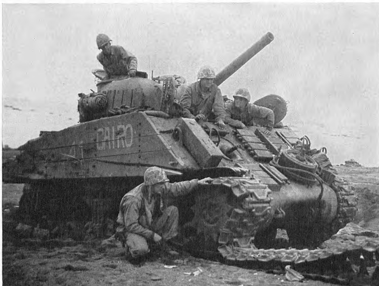
THIS SHERMAN TANK was disabled by a land mine and five hits by Japanese artillery but the crew escaped uninjured. Note heavy planking on side to protect against magnetic demolition charges.
