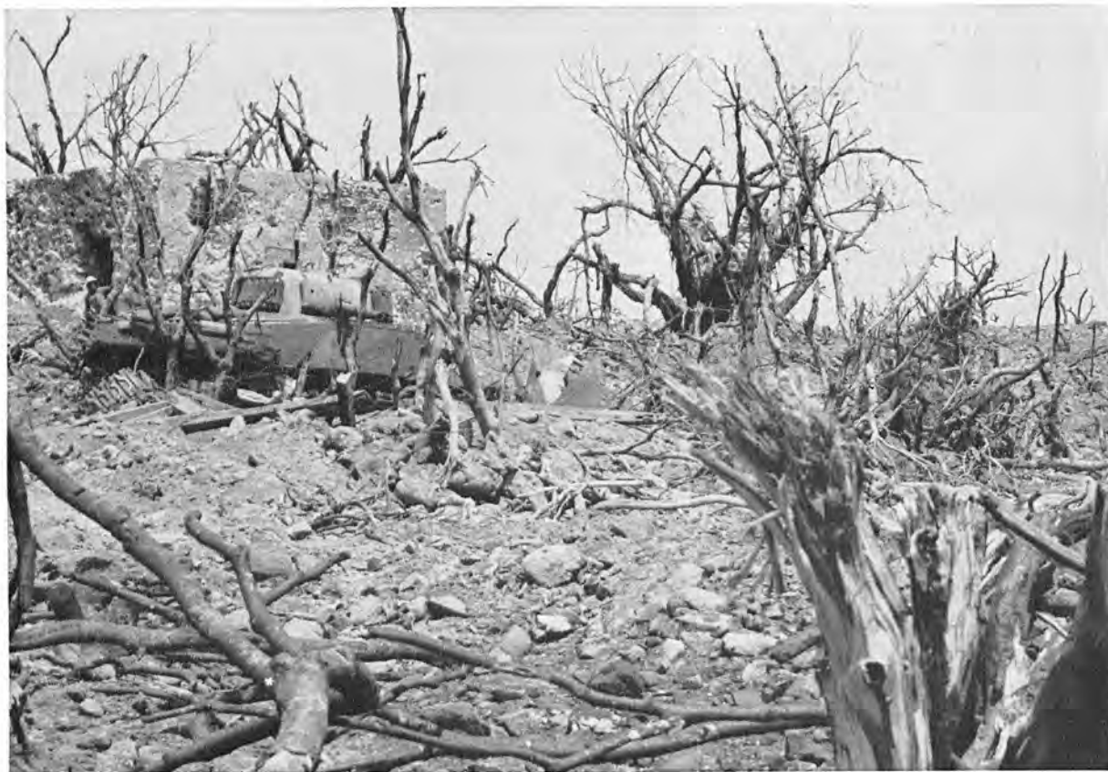
HUGE CONCRETE COMMUNICATIONS BLOCKHOUSE near Turkey Knob. This installation withstood days of direct assault by flame and gun tanks. Sherman next to blockhouse is disabled.
