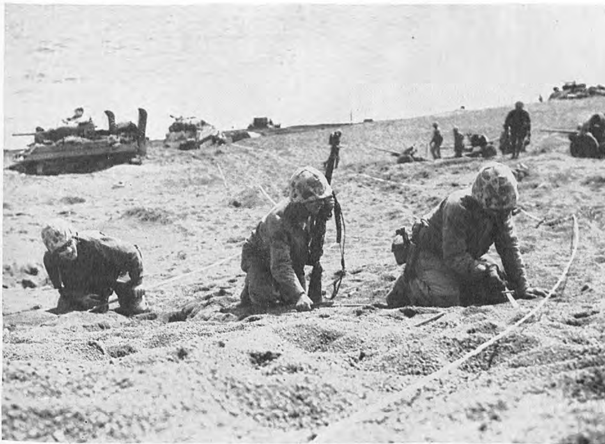
MARINE ENGINEERS in one of their most ticklish operations. Before supporting vehicles could move inland lanes had to be cleared through mine fields. The white tapes mark the safe path through the field.
