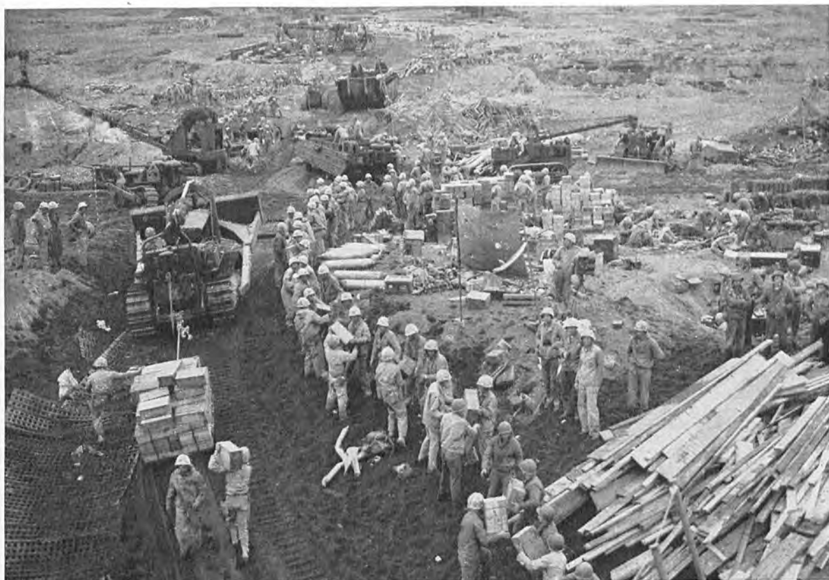
SHORE PARTY PERSONNEL used heavy cargo-handling equipment to keep supplies moving forward. This photo, taken from bow of a landing ship, shows cranes and tractors at work. Note Marston matting road at left. Human conveyor belt expedites the unloading of lighter packaged items.
