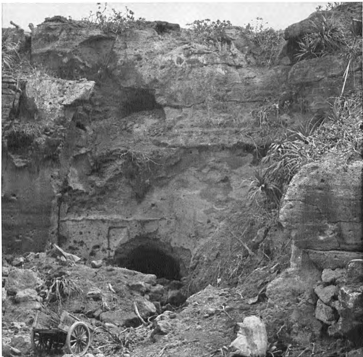
NAVAL GUNFIRE caused landslide which partially blocked entrance to this cave in cliffs above northeastern shore. 3d Division units held positions along top of these cliffs and outposted the beaches as they waited for the 5th Division to advance northward.
