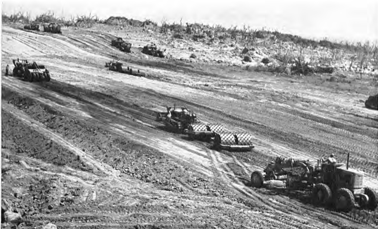
REHABILITATION AND EXTENSION OF THE AIRFIELDS was given high priority. Seabees are shown operating rollers, graders, and huge front-dumping scrapers as they lengthen the east-west runway of Airfield Number 2. (AF Photo)
