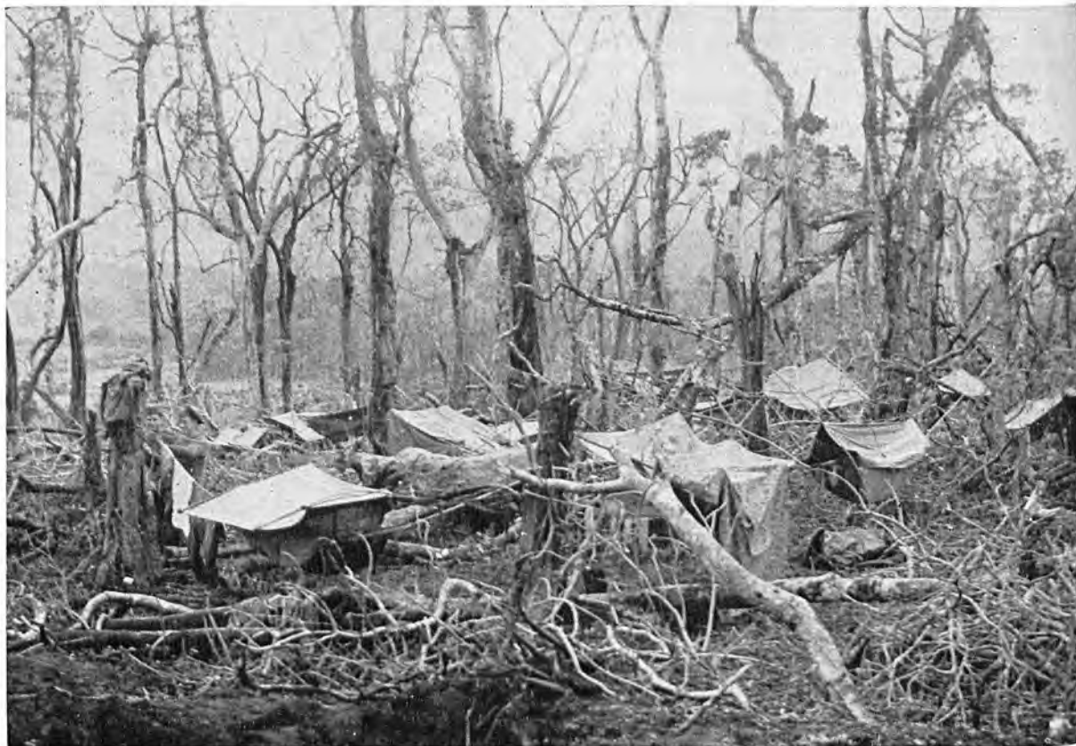
JUNGLE HAMMOCKS were tied to whatever trees were available. This is the Division CP area during an early phase of the operation.
