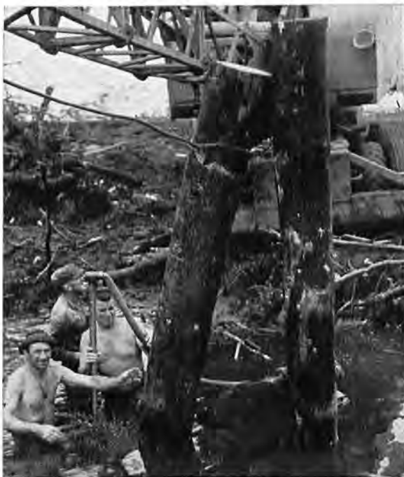
A JET OF AIR AND WATER helped the Seabees place bridge pilings in New Britain streams.
