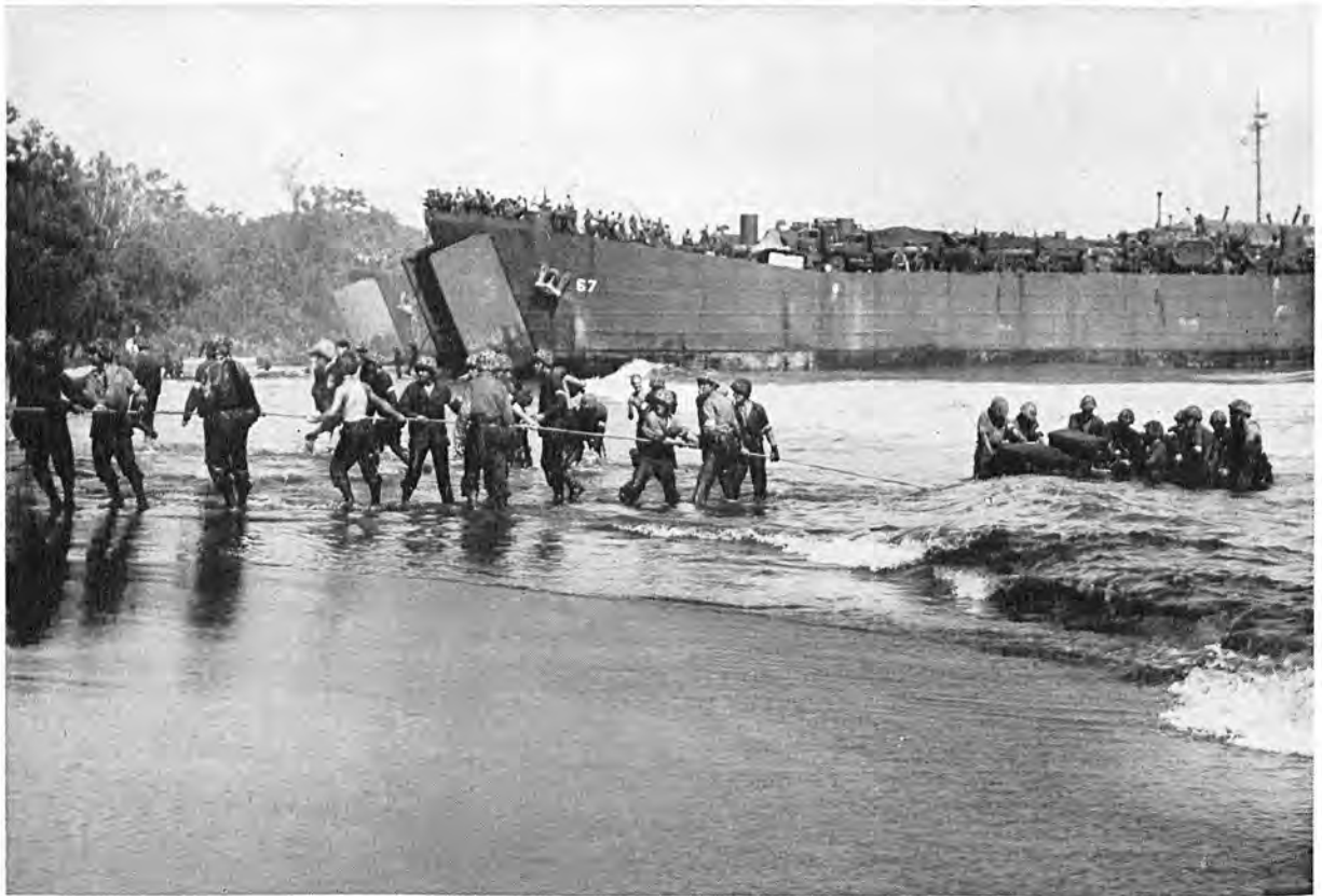
BEFORE THE SANDBAG RAMPS were built, motor vehicles had to be pulled onto the beach.
