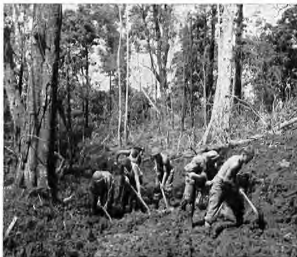
IT TOOK A LOT of work to get the roads in condition.
