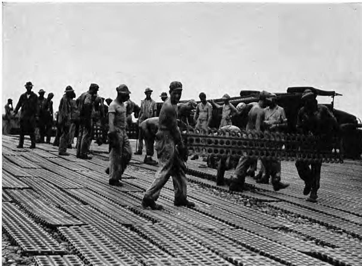
IT TOOK A LOT OF MATTING to get the Gloucester airstrip in usable condition.
