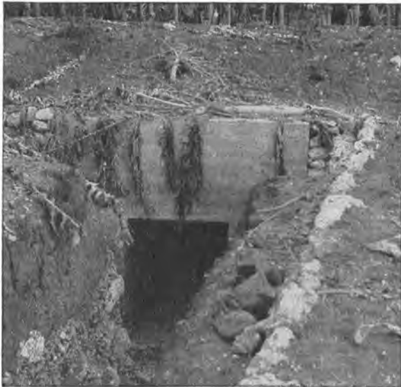
STORAGE VAULT for 120mm dual-purpose gun ammunition. Powerfully constructed positions such as this would have been more common at Saipan if Japanese had not been hampered by a shortage of cement and other materials.
