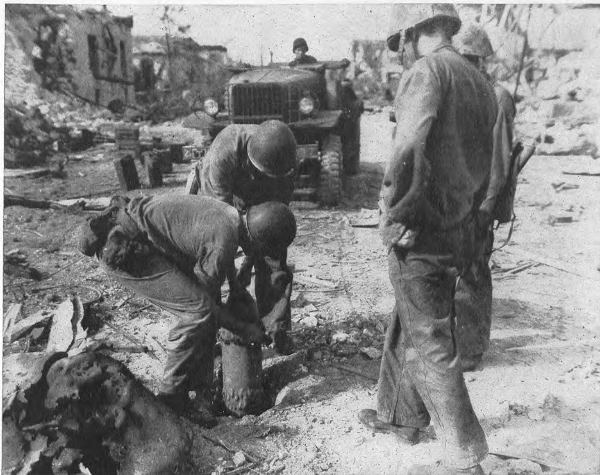
AERIAL BOMBS were extensively employed as land mines by the Japanese. Buried with noses protruding above ground, the bombs could be set off by almost any United States vehicle. This 123-pound bomb was found in Garapan.
