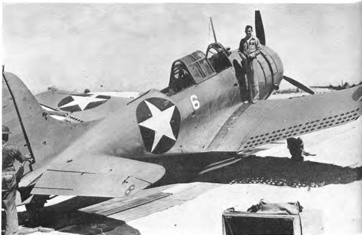
"MY PLANE WAS HIT SEVERAL TIMES," summarized 1st Lt. Daniel Iverson, Jr., in describing the attack by Marine SBD's on the carrier, Akagi . Iverson's dive bomber, shown here, sustained more than 259 counted hits, including one which shot his throat microphone off the pilot's neck.
