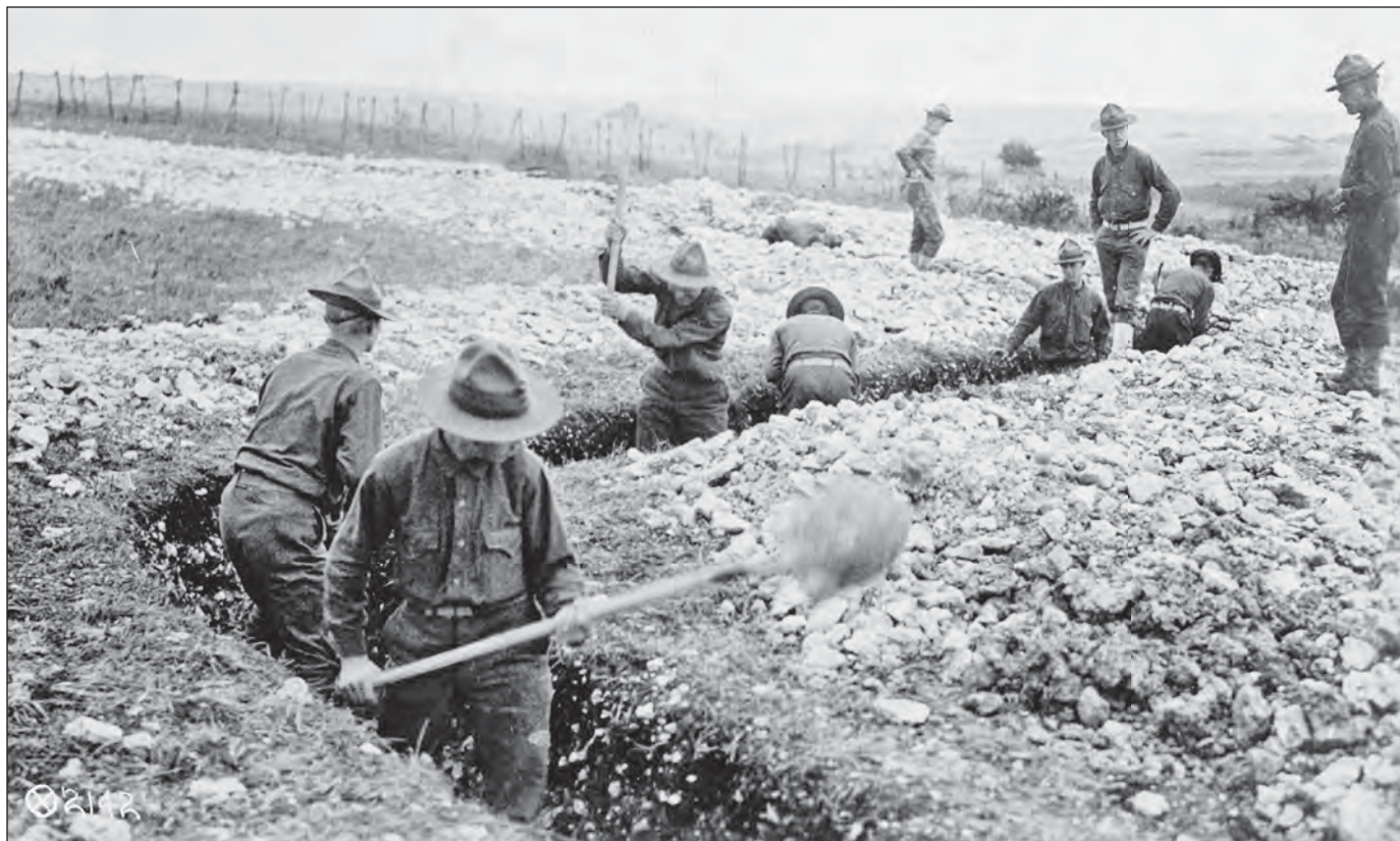
Library of Congress, United States Army Signal Corps Marines in France dig trenches during training for battle.
