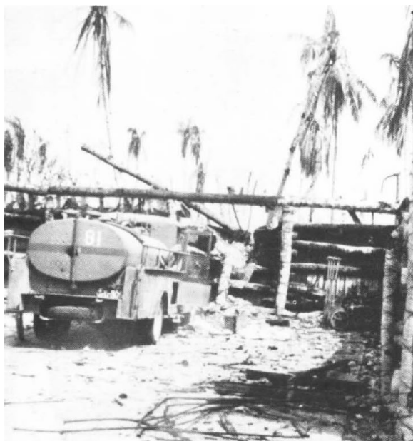
This ground-level photograph identifies the truck in the revetment (above) as a water truck, rather than a gasoline tanker. It also clarifies construction details of the coconut-log-and-coral aircraft revetment.
