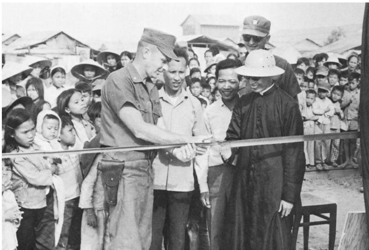
Cdr W. W. DeGroot III, Commanding Officer of Mobile Construction Battalion 58, cuts the ribbon for the 1967 opening of new duplex homes built in the hamlet of Phuoc Quang by the Vietnamese with assistance from the Seabees after a fire left many people homeless. Chaplain R. E. Blade, Civic Action Officer of MCB-58, is in the background.
