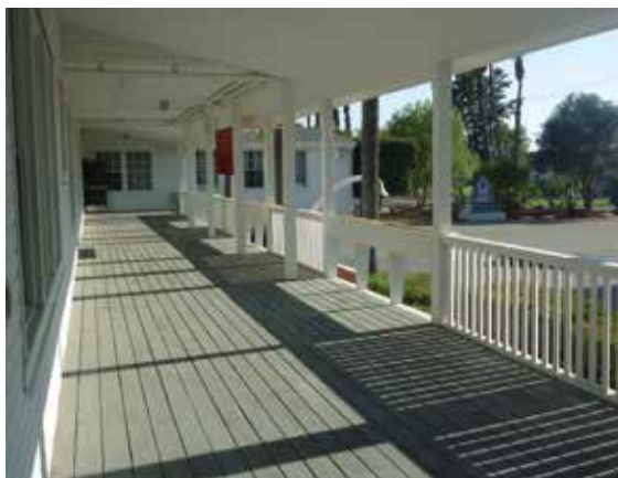
The porch railing of the 1st Marine Division Headquarters has been restored to handrail height.
