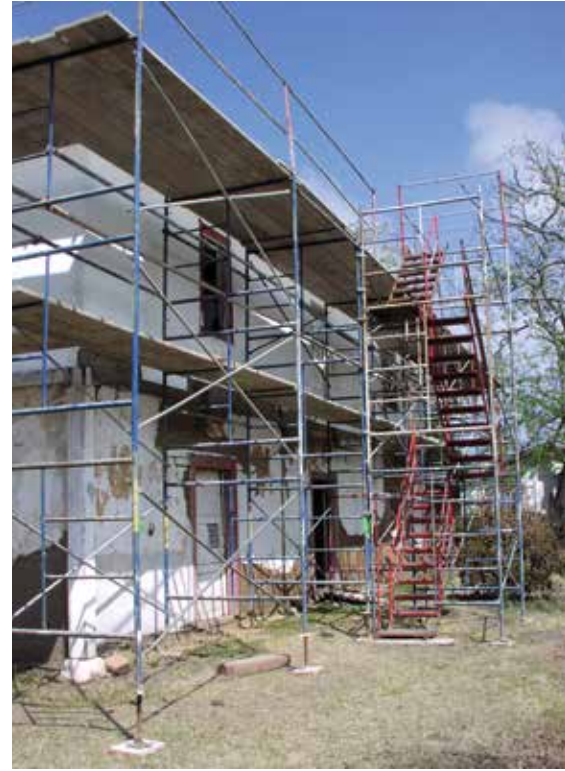
Restoration work on Las Flores Adobe began in 2002 by the University of Vermont with the support of the National Park Service and the U.S. Marine Corps. Surviving plaster was cleaned, and wholesale plaster loss was replaced in kind. New layers of limewash were applied where needed. The National Park Service completed structural stabilization of the main house in 2004. MCB Camp Pendleton Archives
