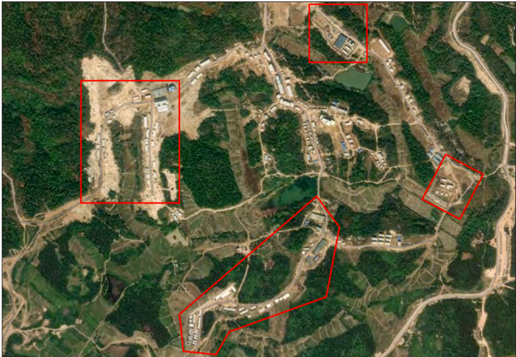
Figure 5. Sanjie Training Base MOUT facilities under construction
