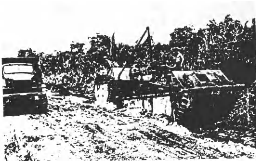
Figure 18. Maintenance in the field took place under difficult circumstances. The engine is being removed from the forward vehicle.
