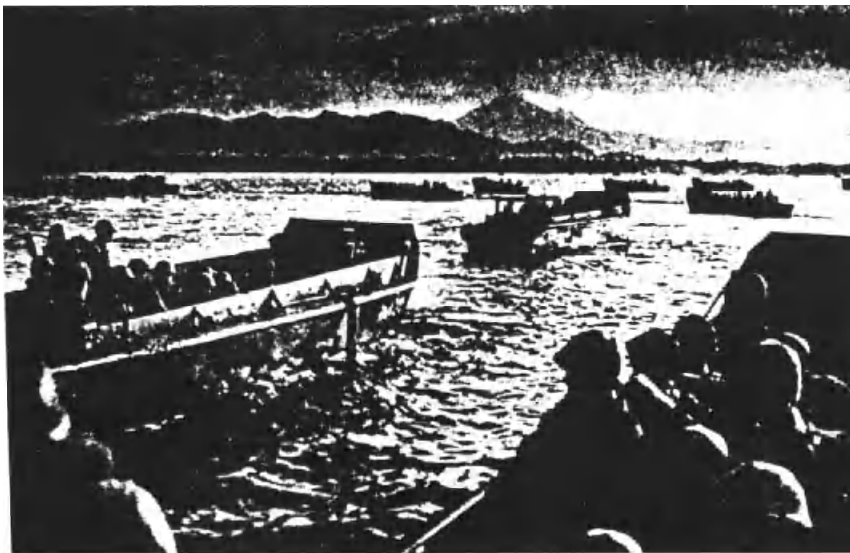
Figure 23. The Landing Craft, Vehicle, Personnel (LCVP). This craft, derived from boats designed for trappers and oil drillers of the lower Mississippi by Andrew Higgins, was the standard landing craft of all theaters of World War II and remains little changed to this day.
