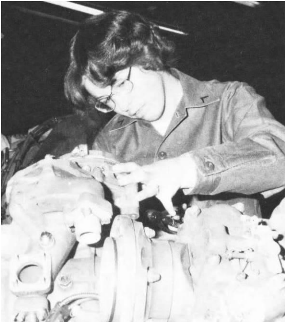
PFC Katie J. Dixon, H&MS-32 mechanic, safety wires the fuel control of an A-4 Skyhawk power plant in the squadron's powerplant section, Marine Corps Air Station, Cherry Point, North Carolina, in 1977.
