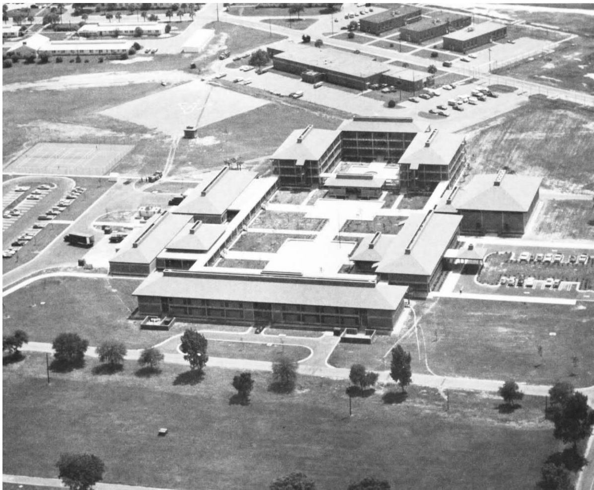
A 1975 air view of newly constructed woman Marine recruit complex at Parris Island.
