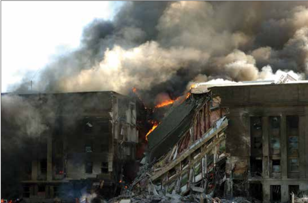
At 0957, the Pentagon's exterior wall collapsed above where the airliner impacted the E Ring. Temperatures from the fire were as high as 1,000 degrees Celsius. Courtesy of the National Archives, photo no. 330-CFD-DM-SD-02-03902.
