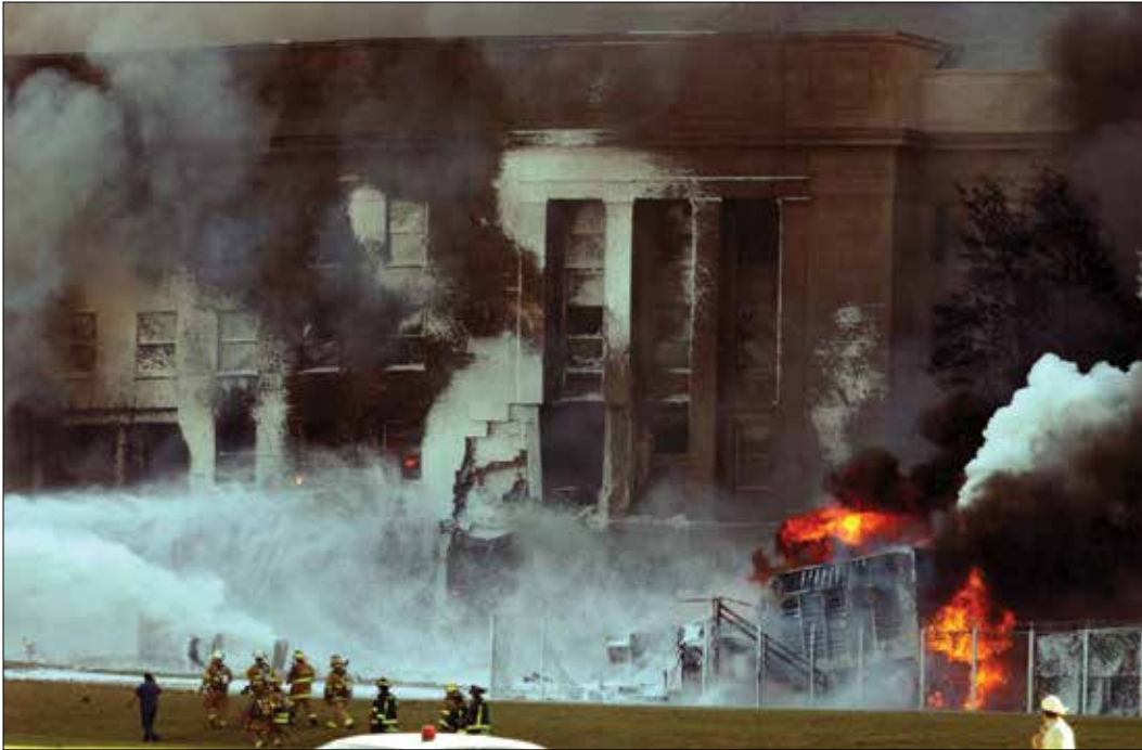
The E Ring exterior minutes before a large part of the wedge collapsed on top of where American Airlines Flight 77 crashed into the Pentagon. Note the cracks in the limestone façade.
