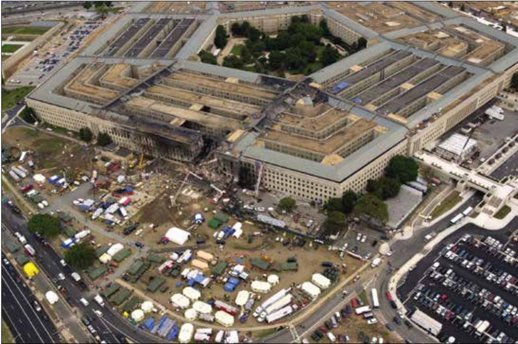
The impact point on the exterior E Ring wall. Note the uniqueness of the Pentagon's structural design, with its rings and corridors, which compartmentalized the destruction and fire. Courtesy of the National Archives, photo no. 330-CFD-DF-SD-02-09101.
